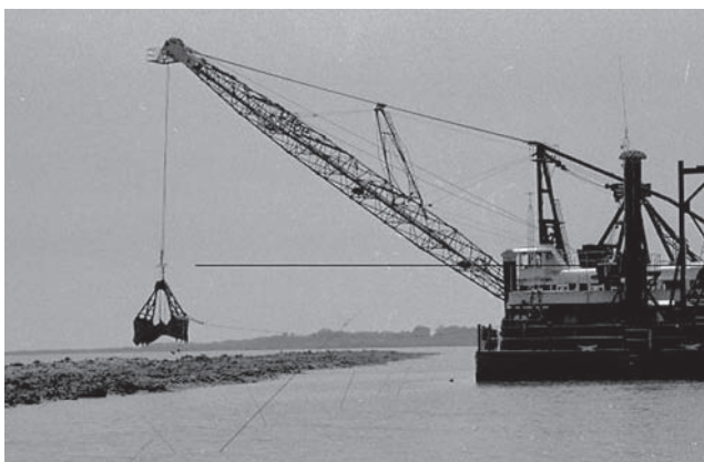
Figure 12: Constructing Terraces to Trap Sediment in Open Water
